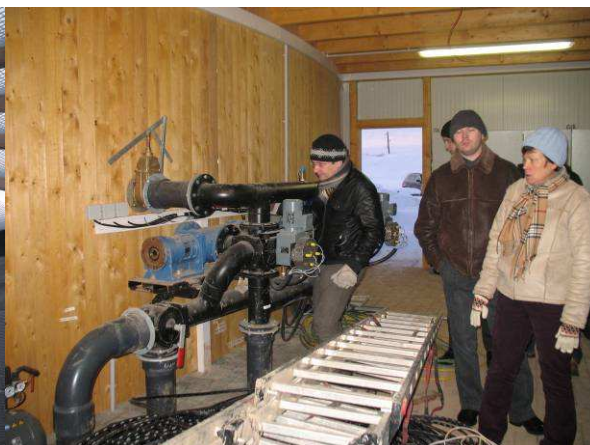
Fig.42. Training participants at the pumping station of “Krūmiņi” biogas plant
