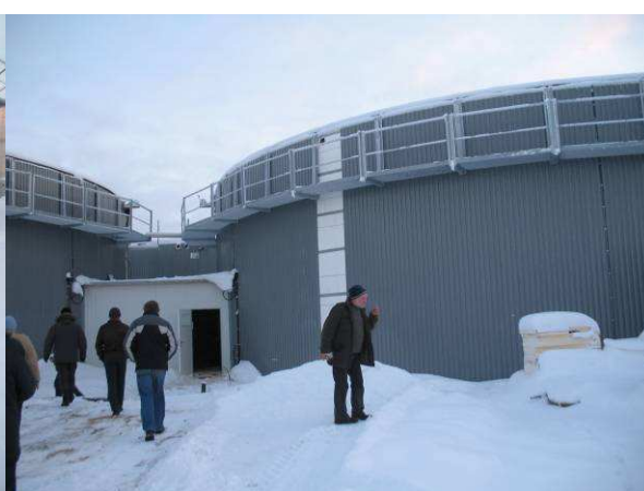
Fig.40. “Krūmiņi” biogas plant in construction
