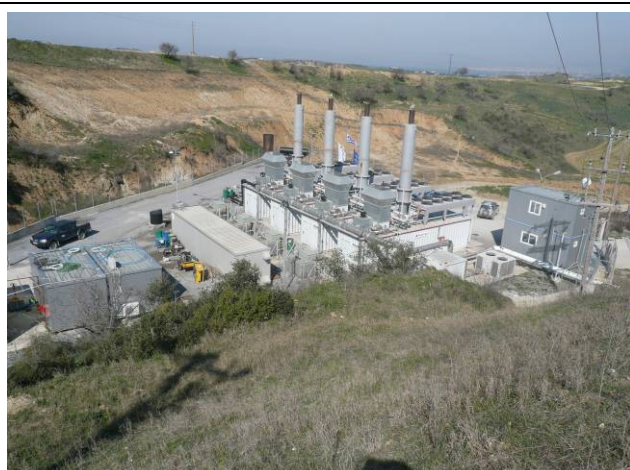
Photo 5: General view of the biogas plant
