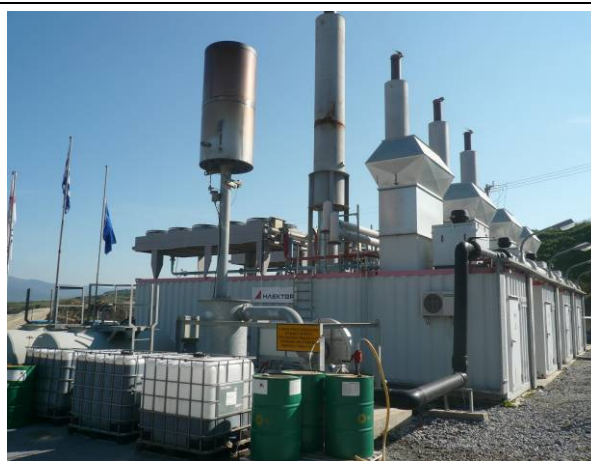
Photo 4: The biogas plant and the flare
