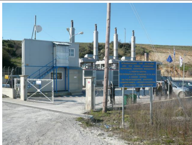
Photo 1: Visit to the biogas plant in Tagarades
