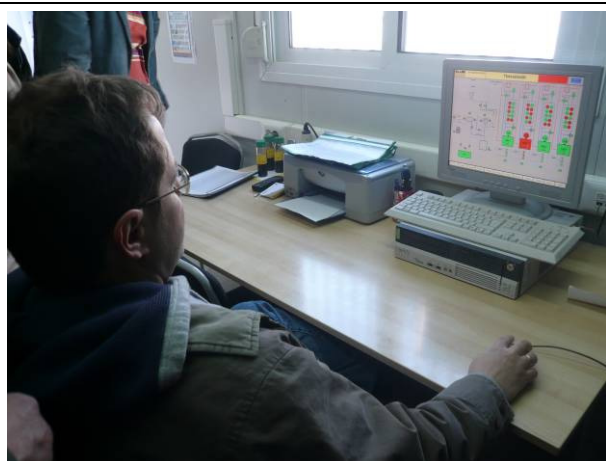
Photo 3: Biogas plant control room
