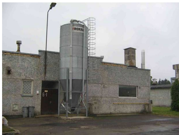
Chicken shed with natural gas boiler
