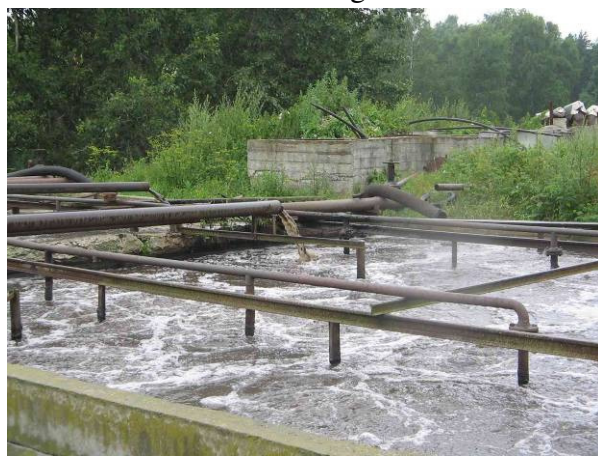
Local wastewater treatment plant
