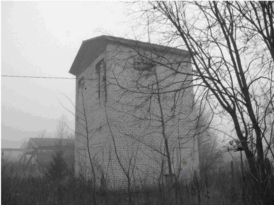
Fig.8. Existing electricity transformation station
