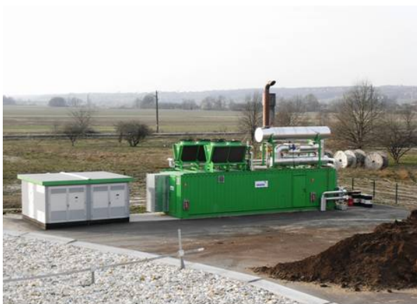
Figure 25. CHP unit seen from atop of a digester, dehydrated digestate can be seen in front
