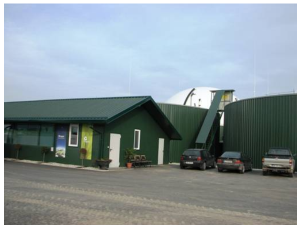
Figure 26. Biogas plant in Dobrovnik is one of the most modern one and it shows also through its exterior
