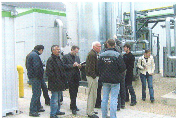
BiG>East Study tour to the first biogas plant in Pliening, Germany, which feeds biomethane into the national gas grid
